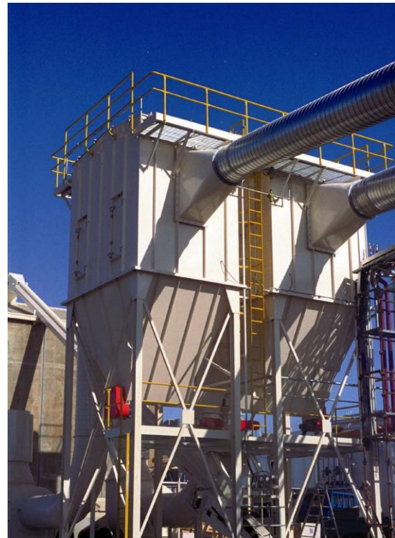
Wood mouldings twin Pulse Jet Filters complete with incline tubulator discharge to silo
