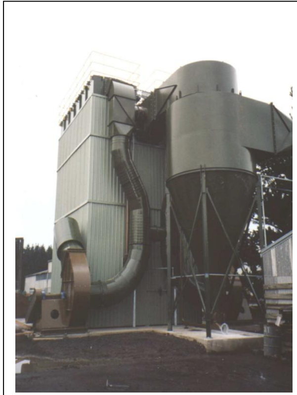
McKechnie metals high temperature smelter fume Pulse Jet Filter complete with grit arrestor
